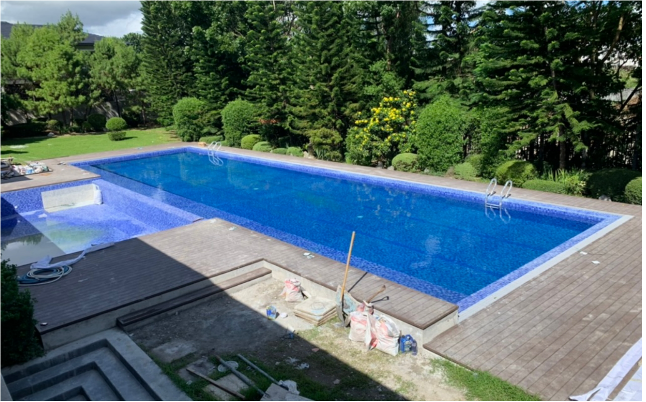
SWIMMING POOL REHABILITATION STATUS PHOTO AS OF NOVEMBER 2022
